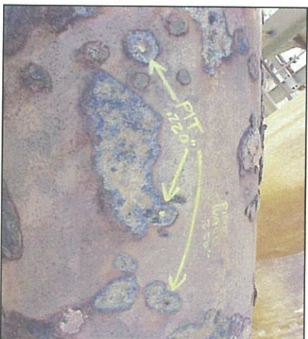
Fig. 2 – Surface preparation as shown is generally unacceptable. In cases where the pipe cannot be properly cleaned, it should be noted that the final ultimate properties of the composite layup may be compromised (such as bonding to the steel surface).
