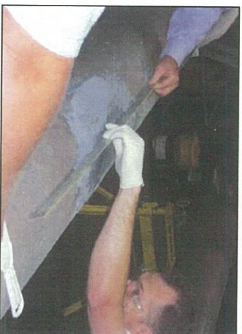
Use a straight edge to confirm evenness
